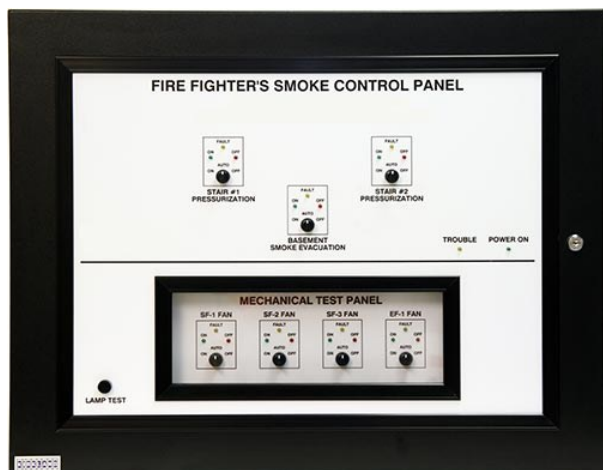
Custom RSF-GR-GP4-FSCS (mechanical test switches only accessible by opening door to panel)
